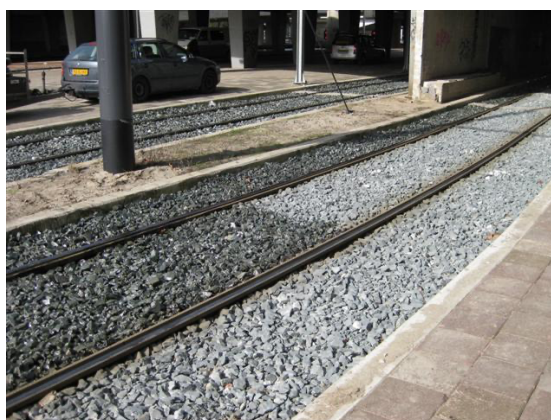
6 – End result reinforced ballast
