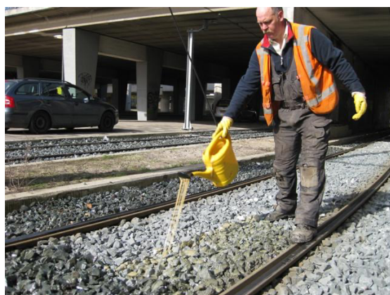
5 – Distribute mixture with watering can over ballast
