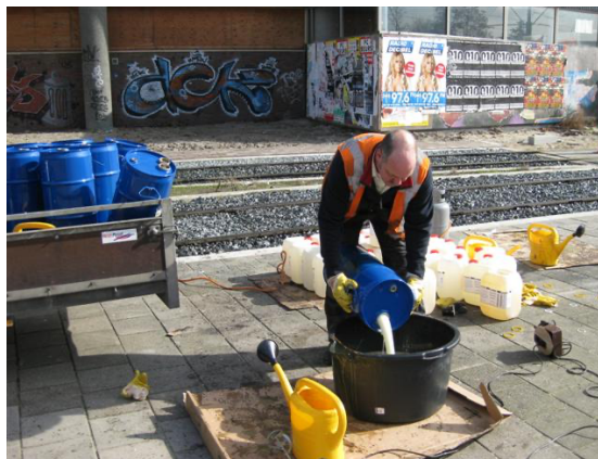
2 – After heating, pour PUR into mixing container
