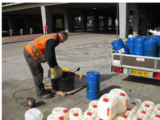
3 – Adding the hardener to PUR
